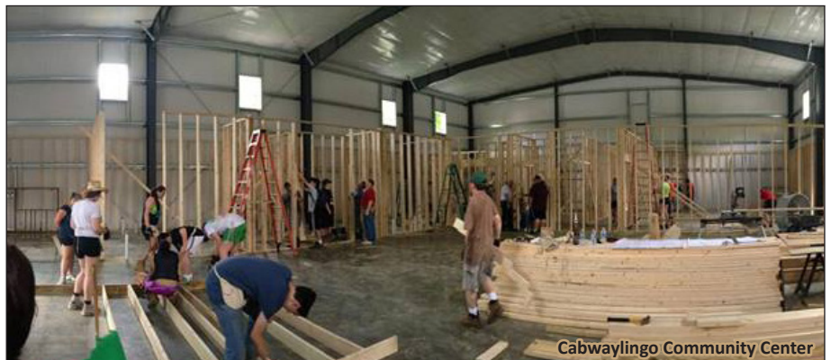
Cabwaylingo Community Center
